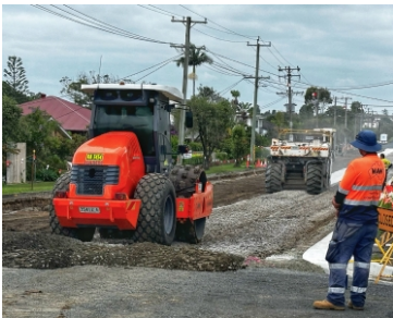
Potholes finally fixed Accepted Wanda Amos
